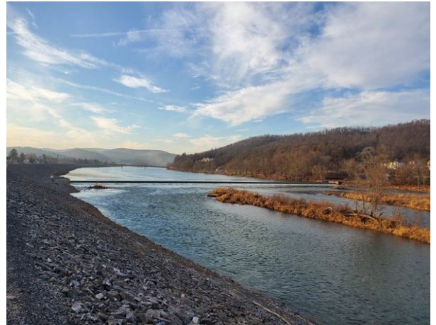
Lock Haven Low Head Dam
